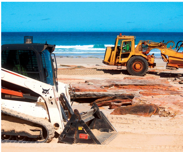
Considerable repair work was undertaken around the Shire following the extreme weather events in 2017/18.
