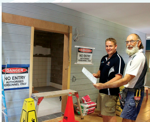
New accessible changing place under construction at BRAC.
