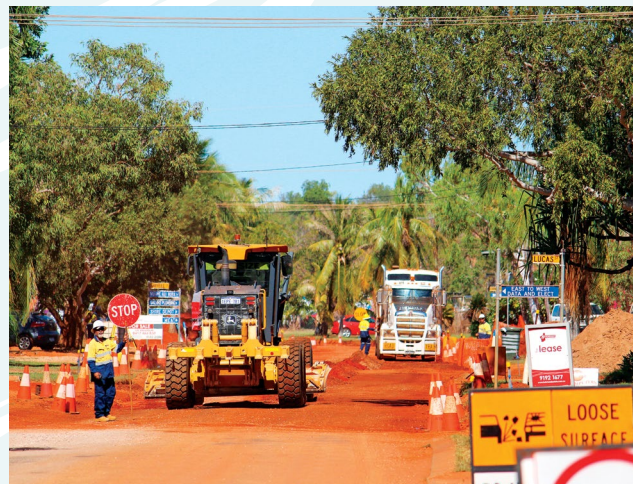
Stage 1 of upgrading Hunter St was completed in 2017/18.
