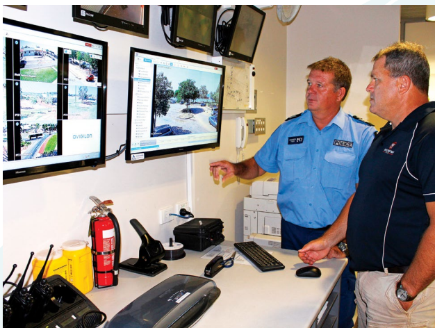
Shire President Cr Harold Tracey inspects vision from newly installed CCTV cameras at Broome Police Station.
