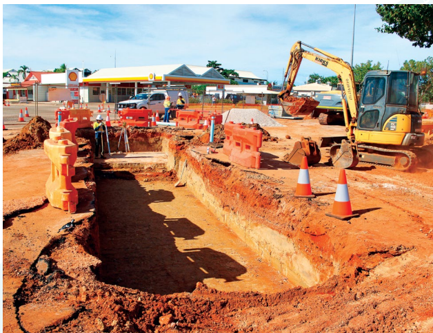
Work is underway on a major upgrade of the Hamersley St – Napier Tce intersection.
