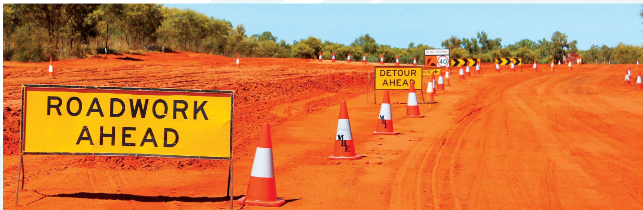
Upgrades to the Crab Ck road under construction.
