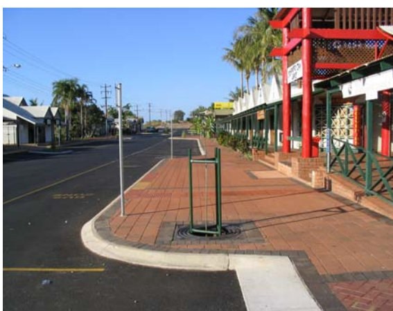
Dampier Terrace, Chinatown – following works
