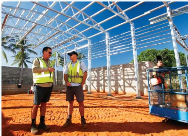
Work on the new Broome Civic Centre neared completion in 2011/12.
