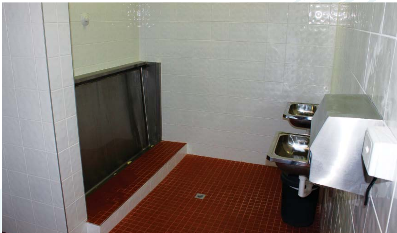
Capital works in 2012/13 included upgrades to ablutions at Town Beach.
