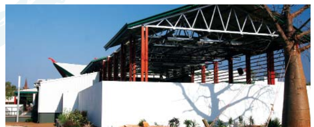
The new Broome Civic Centre.
