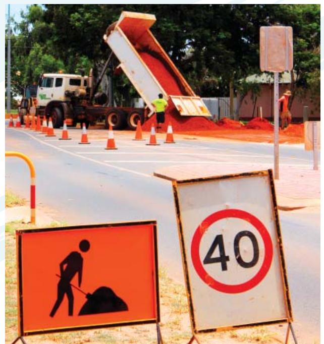
Further changes to Frederick St have improved road safety.
