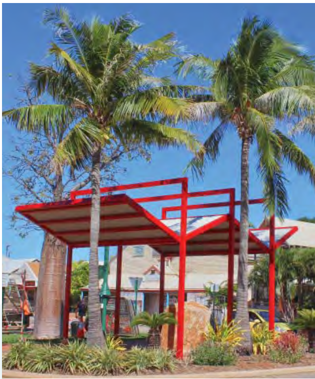
New shade structures going up in Chinatown.
