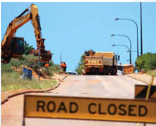
Work to improve road safety at a Black Spot on Carnarvon St.
