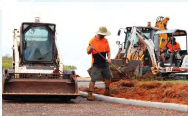
Work underway at the Town Beach boat ramp.
