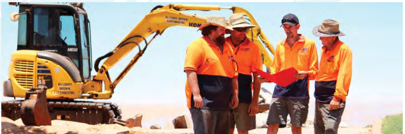
Work on a $500,000 renovation of the Town Beach boat ramp.
