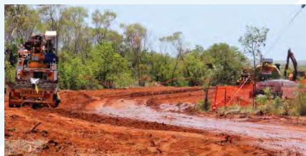
Work on the extension of Lorikeet Dve to Broome Hwy.
