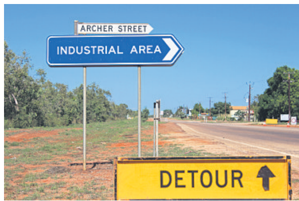
Archer St in the Port Dve industrial area is being rebuilt.
