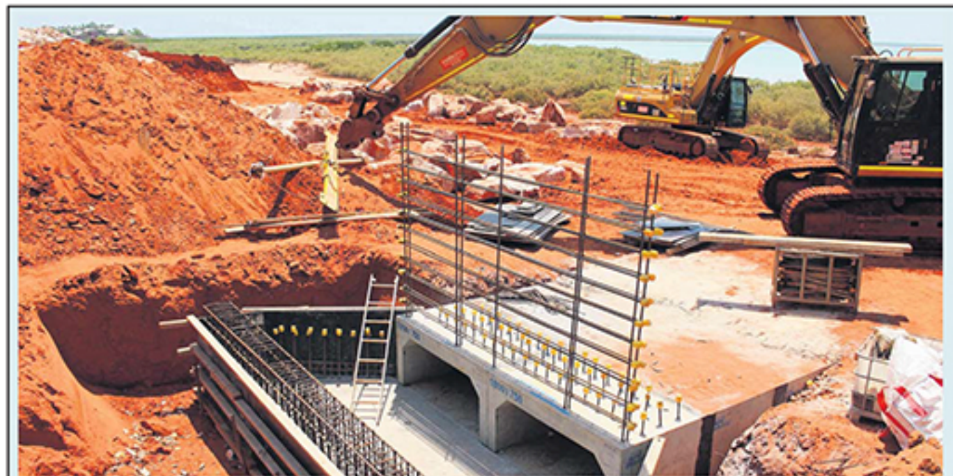
Work on the seawall at Town Beach is progressing with drainage now in place.
