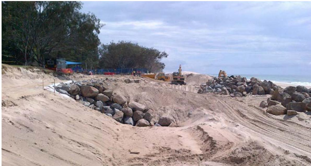
Figure 6.5: Buried Seawall under construction (GCCC 2016)
