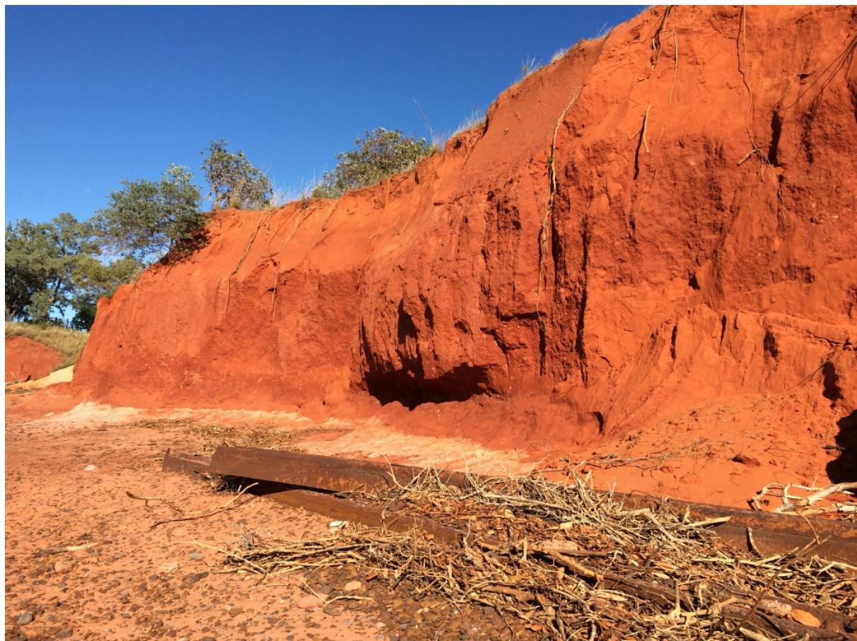
**Figure 6.8: Town Beach eroding pindan cliff with example of undercut cliff base**
