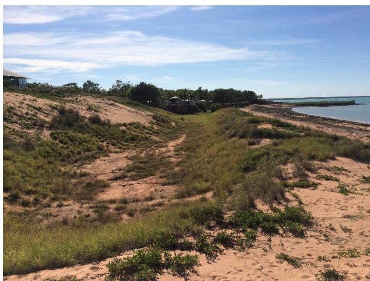
**Figure 6.10: Low Point in dune affecting coastal erosion hazard for properties on Demco Drive**
