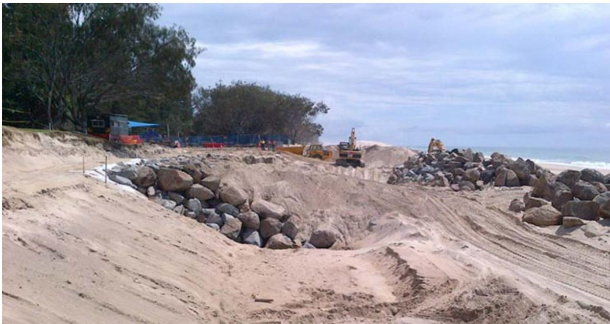
Figure 6.5: Buried Seawall under construction (GCCC 2016)
