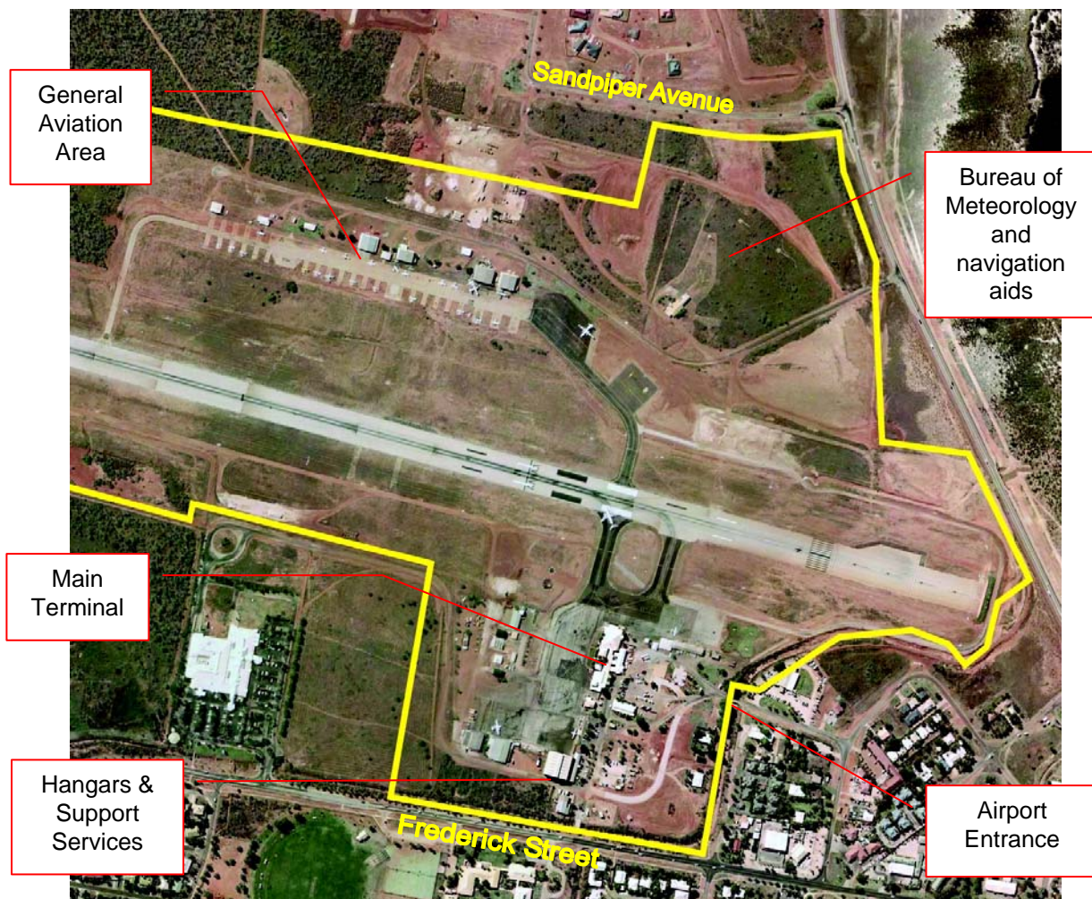
Figure 6 Broome Airport – Eastern End; Primary Use Areas
