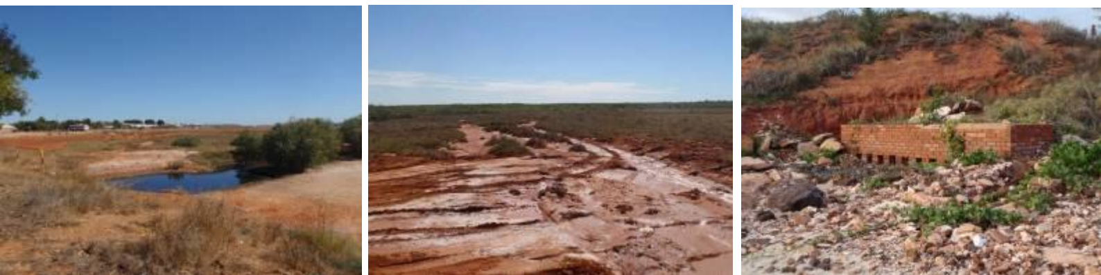
EXISTING DRAINAGE WITHIN BROOME Photo by UDLA
