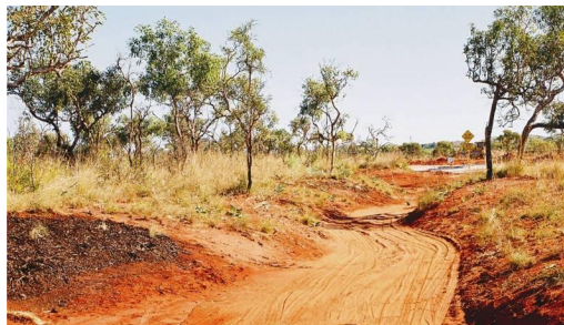
FREE FORM DRAINAGE SWALES – JANUBURU SIX SEASONS, BROOME
