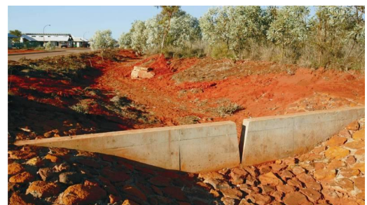
CONCRETE WEIRS– JANUBURU SIX SEASONS, BROOME
