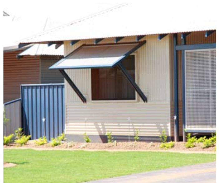
A typical awning, perforations allow breezes to pass through it.
