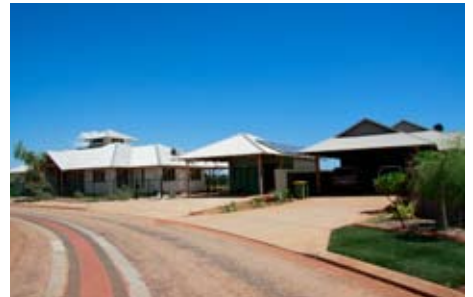
Janubaru Six Seasons. typical street layout with raised blocks, mountable kerb and no footpath. House typically 4-6 m from street edge.
