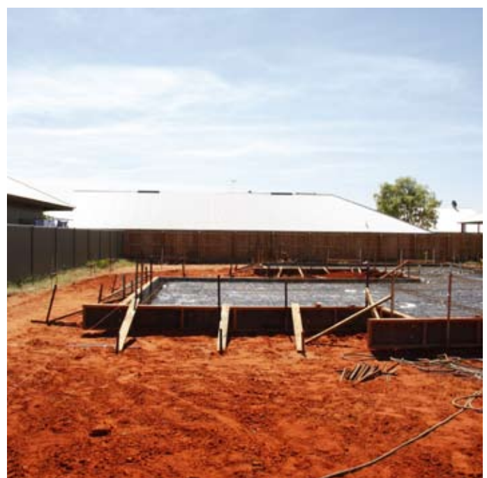
New Broome houses are typically slab on ground.
