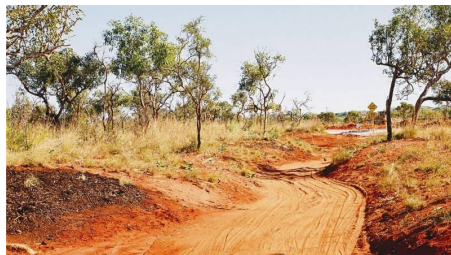
FREE FORM DRAINAGE SWALES – JANUBURU SIX SEASONS, BROOME Swales direct water around significant vegetation and landform Photo by UDLA
