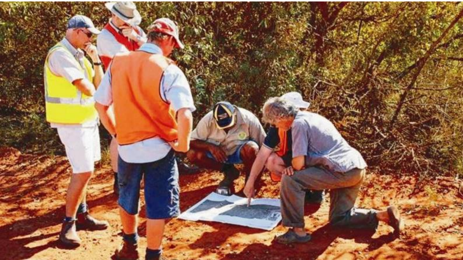
DISCUSSING NEW DRAINAGE SOLUTIONS Photo by UDLA
