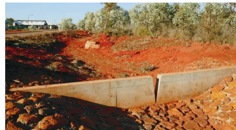
CONCRETE WEIRS– JANUBURU SIX SEASONS, BROOME For water retention and slow release Photo by UDLA
