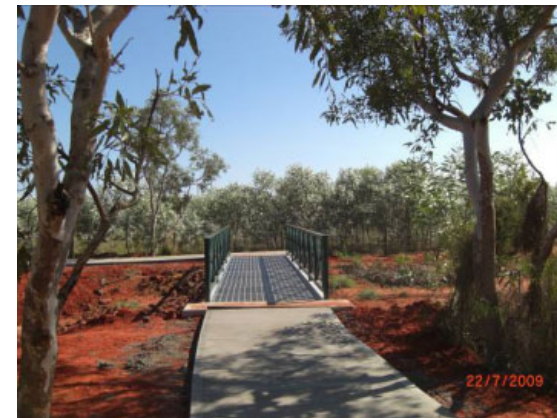
Figure 3.15 Pedestrian Walkway Bridge
