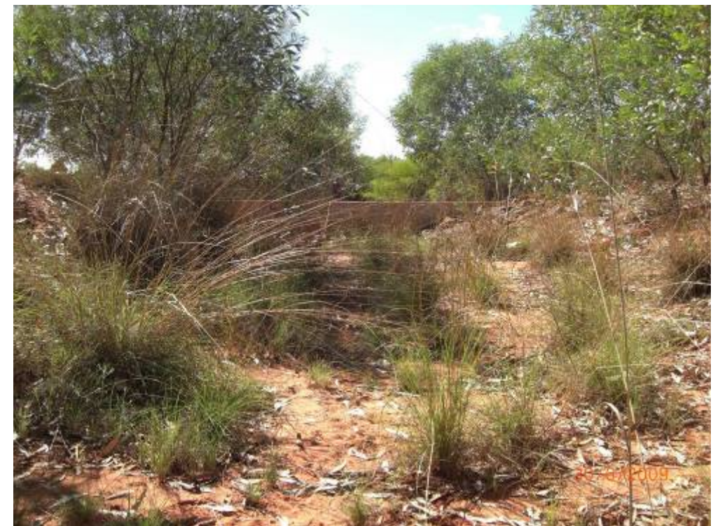
Figure 3.1 Typical Vegetated Drainage Swale with “Low Flow” Notch Weir
