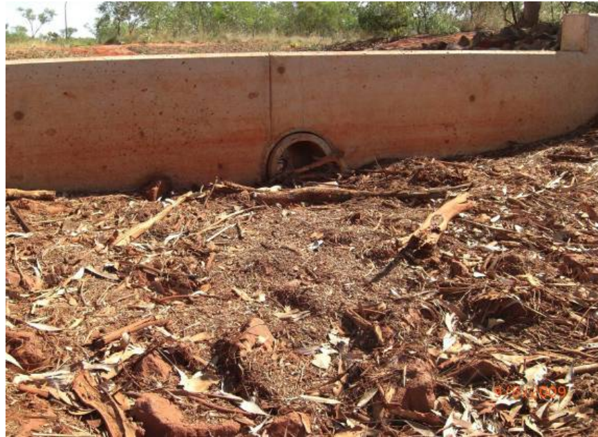
Figure 3.12 Typical Detention Basin Weir with Low Flow Outlet – Upper Catchment
