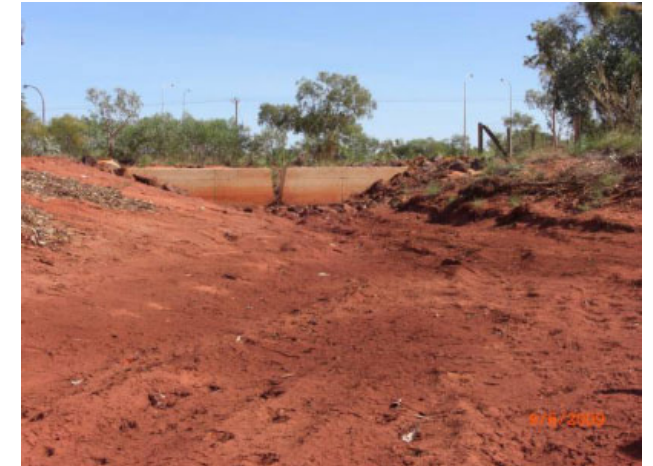
Figure 3.6 Typical Dry/Ephemeral Detention Basin
