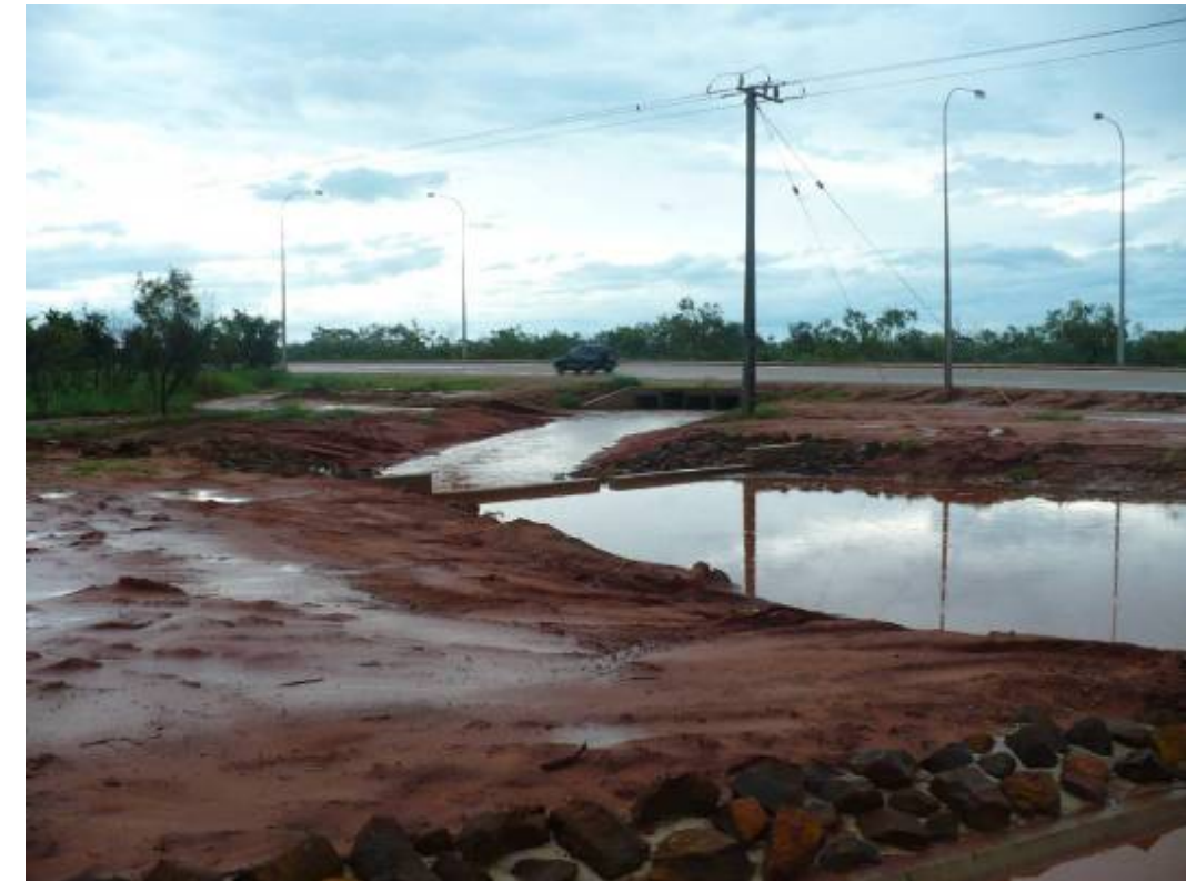
Figure 3.3 Detention Basin, Weir and Low Flow Notch Outlet
