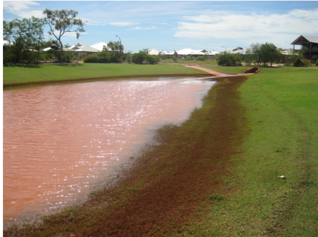
Figure 3.2 Multi-Use Drainage Basin
