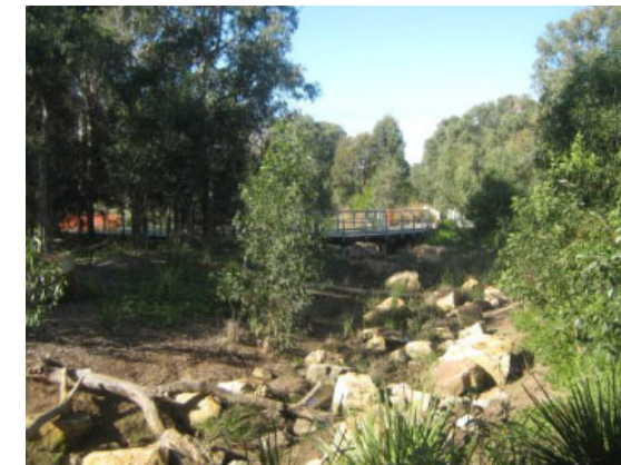
Figure 3.16 Creek and Bridge
