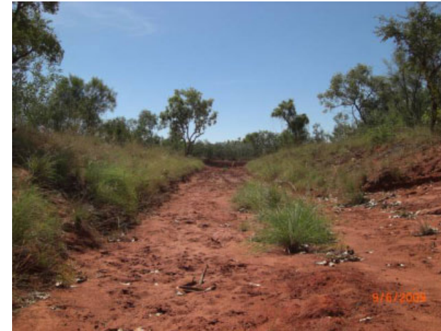
Figure 3.5 Typical Vegetated Swale
