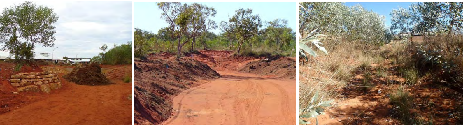
DRAINAGE SWALES WITHIN THE ECC Photos courtesy of UDLA, 2006-2009
