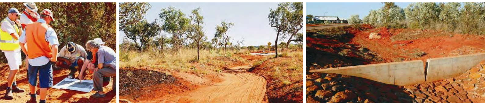
DISCUSSING NEW DRAINAGE SOLUTIONS / FREE FORM DRAINAGE SWALES / CONCRETE WEIRS JANUBURU SIX SEASONS, BROOME Photo by UDLA
