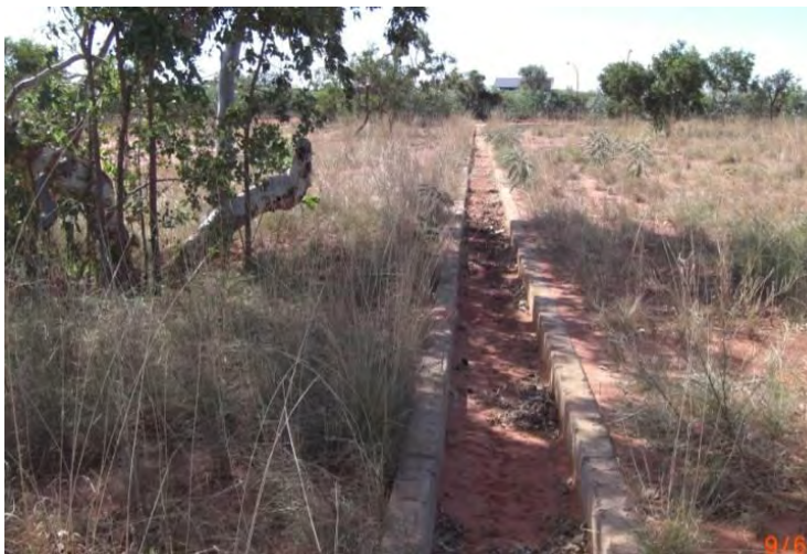
CONCRETE BASED DRAINAGE EASEMENT – JANUBURU STAGE FOUR Photo courtesy of SKM, 2009 Drawing by UDLA, 2008
