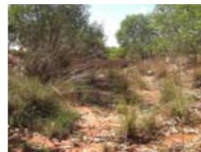
example of a constructed open drainage swale that has been re-vegetated
