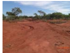
example of a small dry/ephemeral detention basin with weir control - recently constructed
