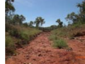
example of an open drainage swale where mulched vegetation has been used on the embankments to encourage re-growth
