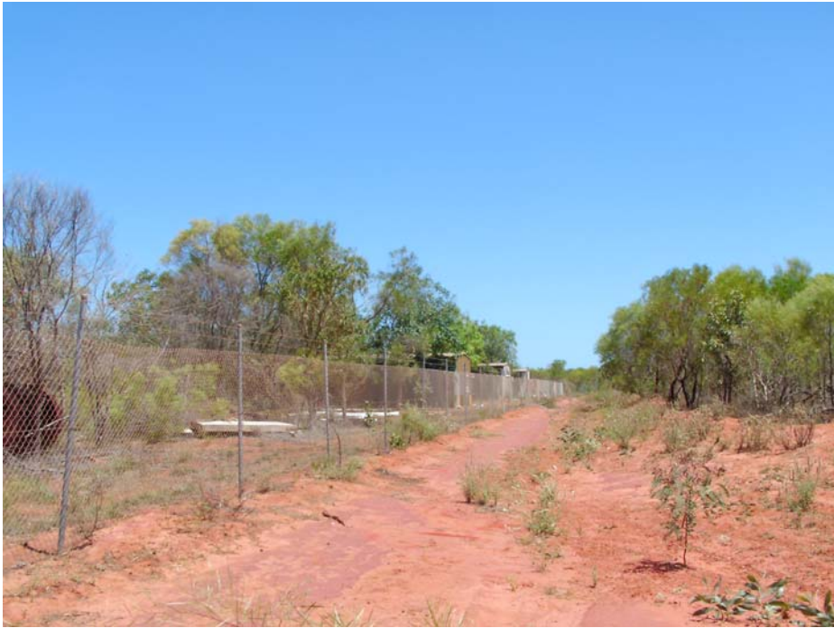
Photo Plate 2 – Drain/firebreak on site perimeter
