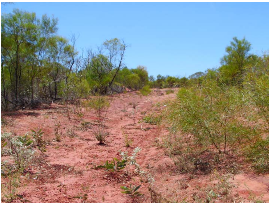
Photo Plate 3 – Drain leading to Fairway Drive
