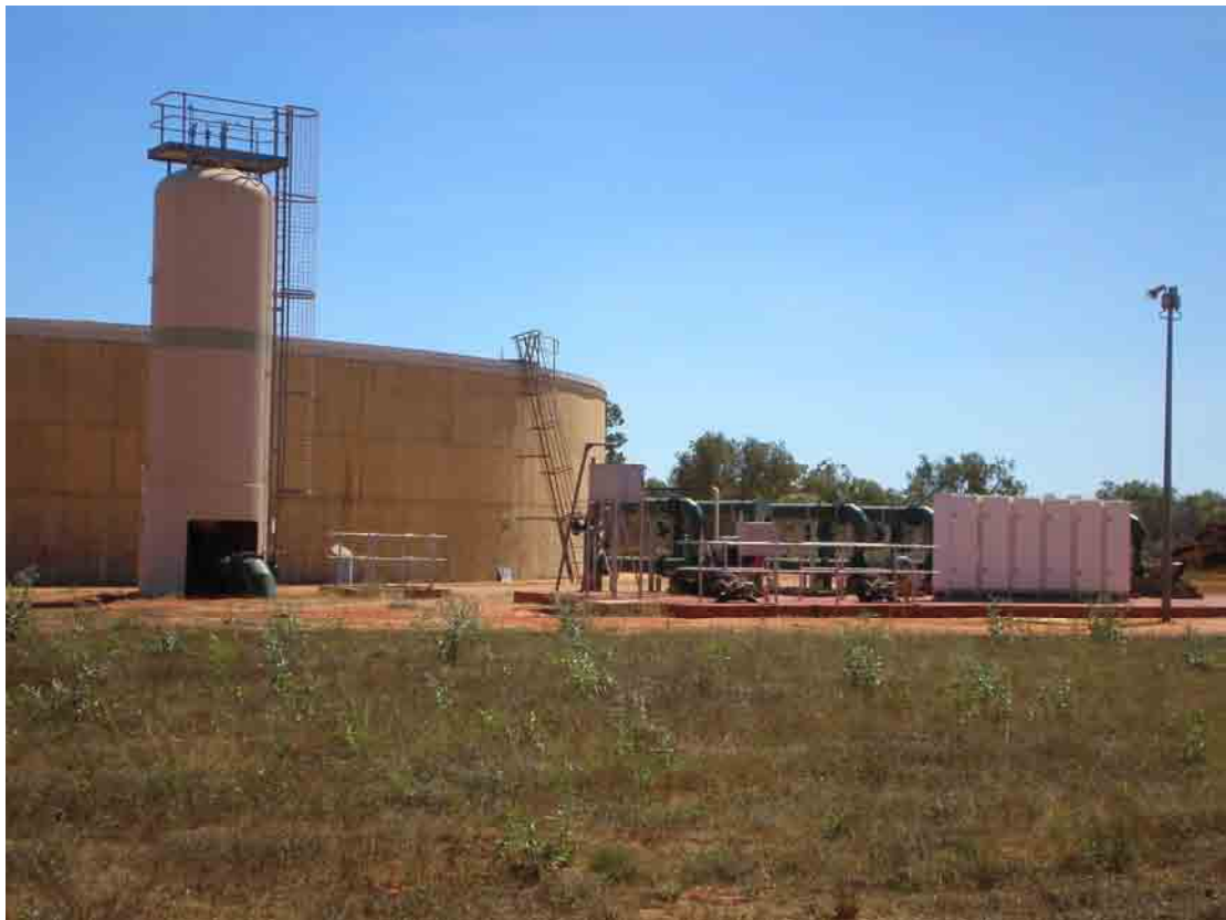
Plate 4: Water Corporation Enclosure – Water Tank and Pumping Equipment.
