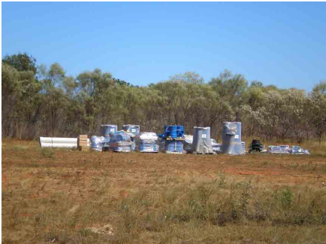
Plate 6: Water Corporation Enclosure – Laydown Area.
