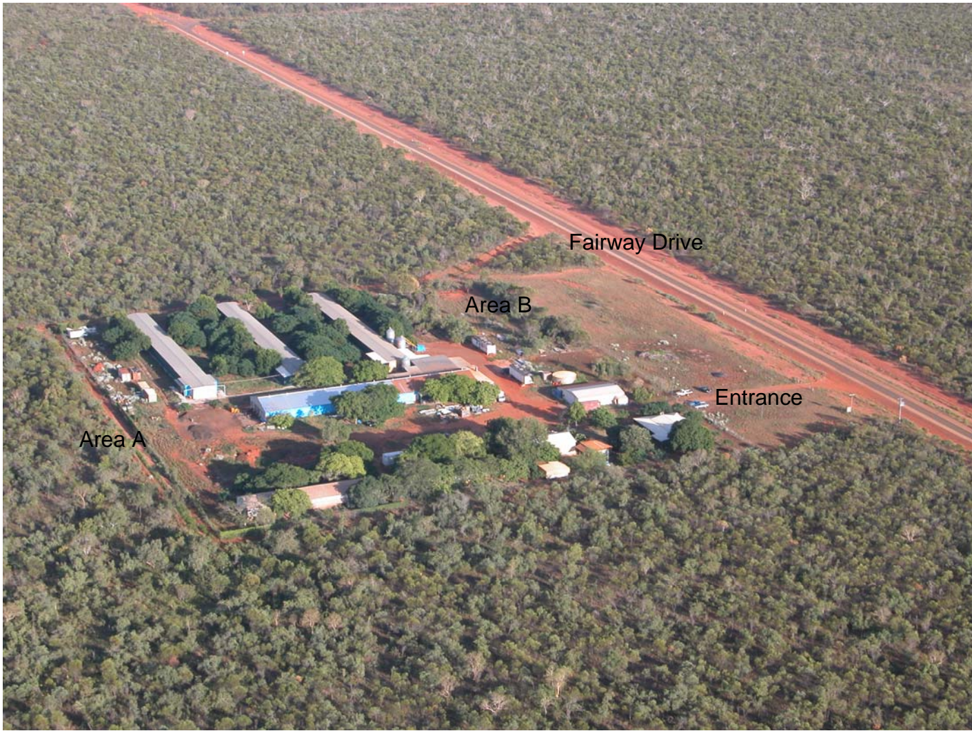
Photo Plate 1: Aerial photograph of the site showing areas where scrap is located
