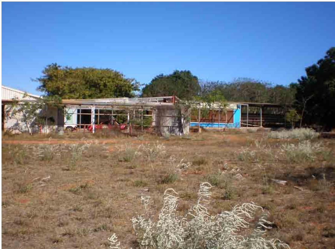
Plate 2: Former Poultry Farm – Unsealed Ground Surface.
