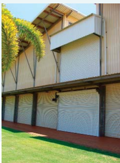
Upgraded roller shutter doors have been installed at the Broome Recreation and Aquatic Centre along with other works to provide a secure emergency centre.
