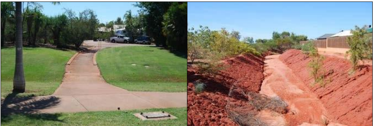
Figure 11: Integration of stormwater into local public open space (left), compared to traditional trapezoidal drains which may lead to erosion, channelling and health and safety issues (right).
