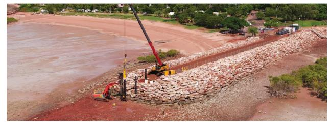
The construction of a new 110m jetty at Town Beach is well underway, with the project on track despite recent wet weather.
