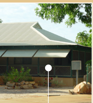
Wide usable verandahs
